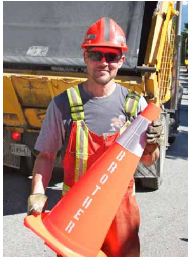
A proper work zone set up is critical for worker safety.
