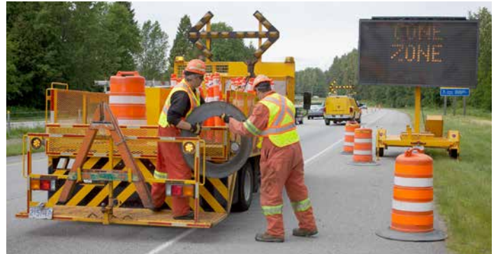
Set up work zone devices in the order that drivers will see them.
