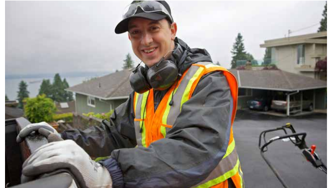
Each road side work zone has its own unique set of hazards.
